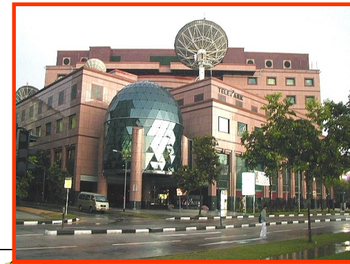
Telepark (Network Hub)
